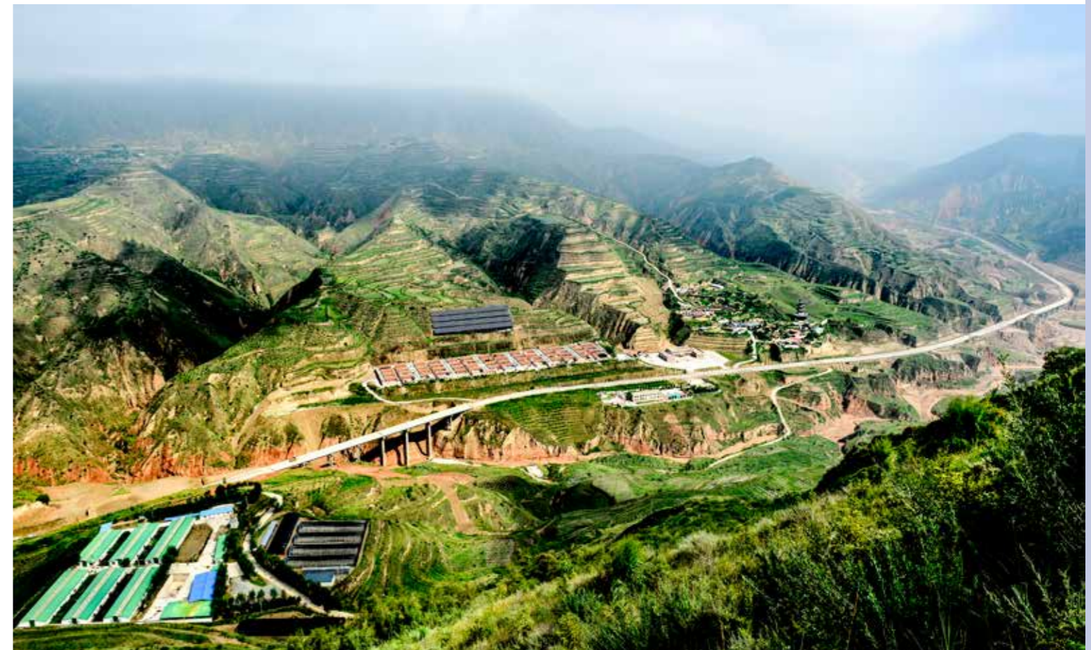
The hardened road to Bulenggou Village, which was built with the assistance of Sinopec
